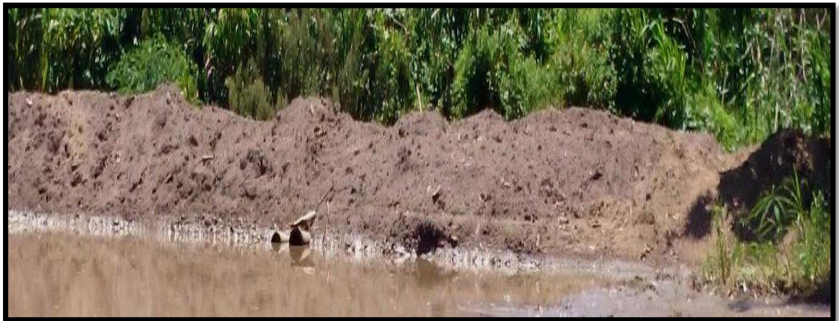
Image 2.3: Example of Temporary sand berm
