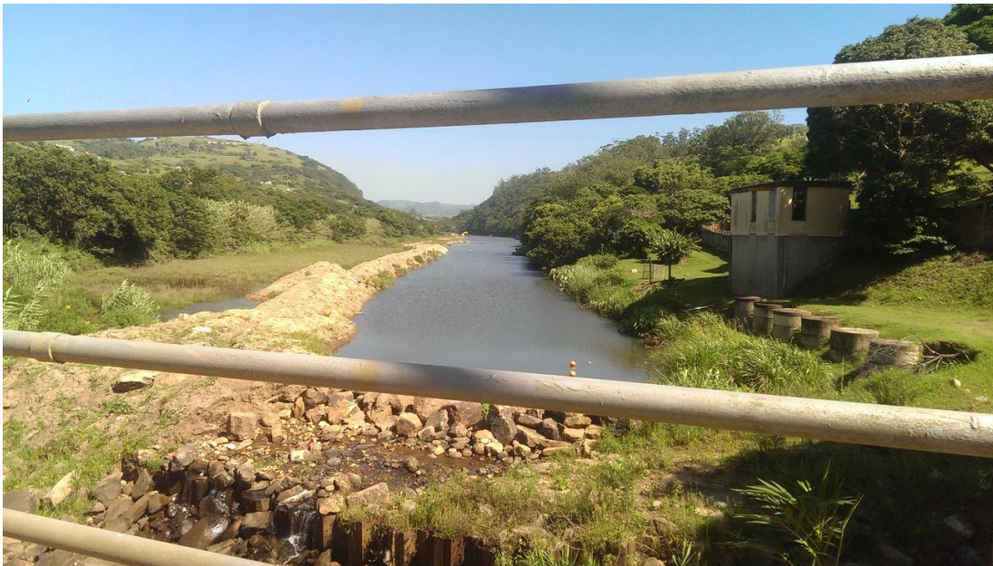
Image 3.5: The Mtwalume Water Works
