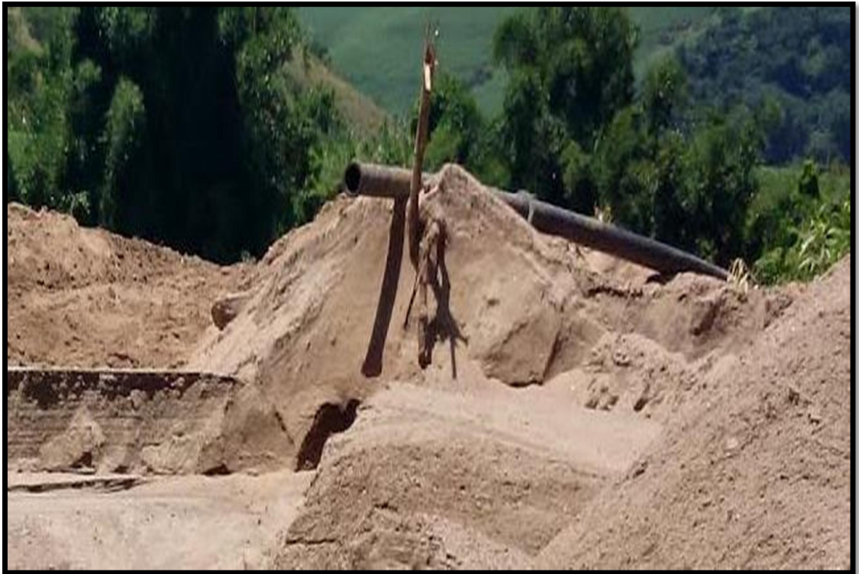
Image 2.4: Example of Pipe outlet into stockpile area
